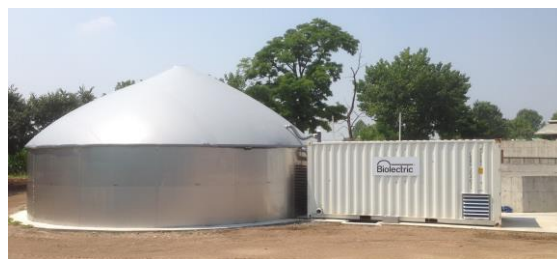
Figure 23: Biogas Installation (Source: Bioelectric, Belgium)
