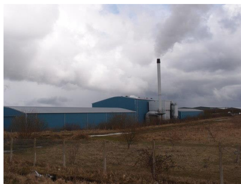
Figure 15: Elean power station
