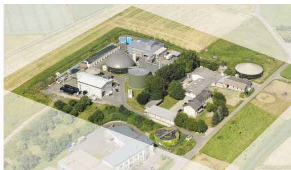
Figure 3: Biowert Biorefinery Plant (Source: https://biorrefineria.blogspot.hu/2016/04/biowert-biorefinery-biorrefineria-verde-green.html )
