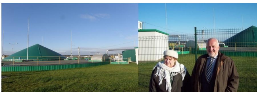
Figure 10: General view of biogas station and a picture with the owner.
