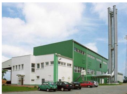
Figure 8: General view of Pisz heating plant,
