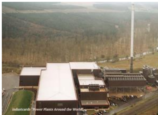
Figure 18: Thetford power station
